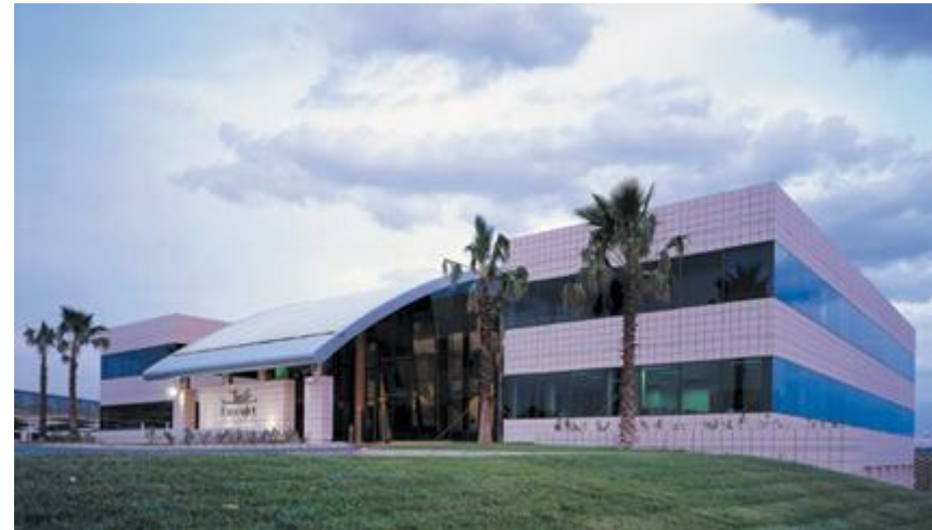
Facilities at Lanseria Airport, South Africa
