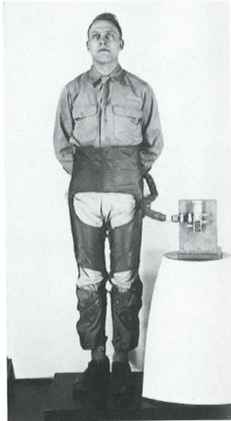
1940s Prototype of a Pneumatic G Suit [Source: McDonnell Aircraft Company]
